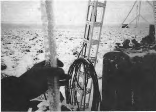
Figure 9: Author illustrates the effect of freezing rain on summer grade navigation towers.
