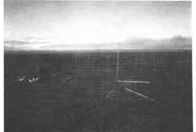
Figure 13: Shore Station Failure due to High Winds on Herschel Island.
