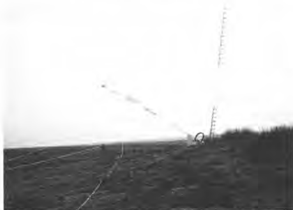
Figure 6: Erecting the Tower.
