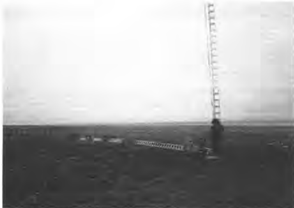
Figure 5: Erecting a 100 Foot Syledis navigation tower.
