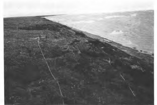
Figure 14: Station Failure due to Bank Erosion.
