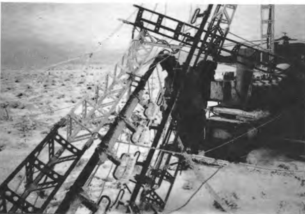
Figure 11: Station Failure due to Ice Load
