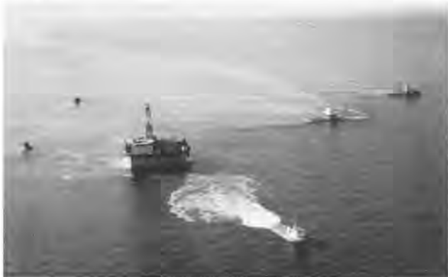
FIGURE 11 MOLIKPAQ BEING POSITIONED OVER THE TARSUOT P45 BERM
